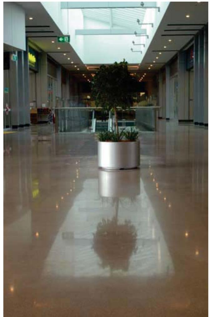
The Hiperfloor™ process transforms already existing concrete substrate into wear resistant, beautiful floors. This reduces the requirements to install other surface treatments.
